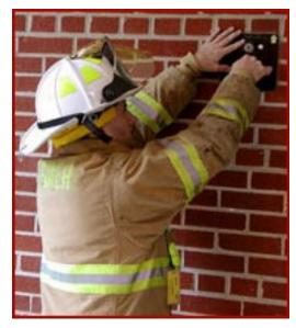
A Knox Box is a small, safe-like, box that attaches to the home or entry door. A key to the home is placed inside the box. The box can only be accessed by a special key that the fire department carries with them at all times. These boxes are very secure as access to the key is limited.
